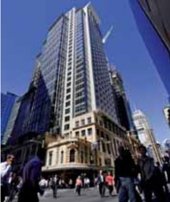
Telstra building, Sydney CBD
